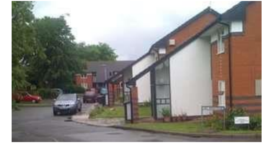
Cae Bracty – proposed individual property flood protection and addition of Smart controls to existing storage tank and pump.
